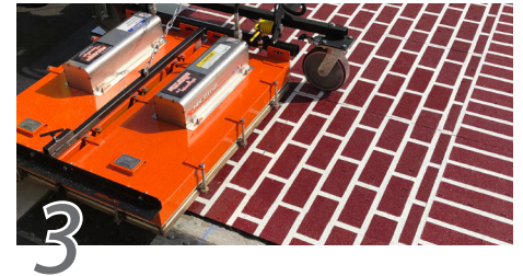
Heat material until sufficiently bonded to the surface
