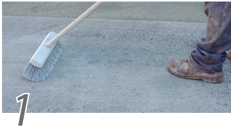
Clear area, remove moisture and apply sealer
